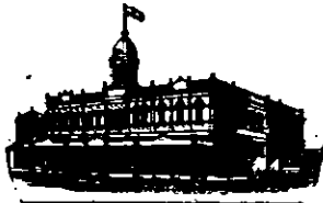
Te Aro House WELLINGTON
