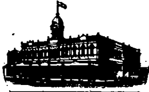
Te Aro House WELLINGTON
