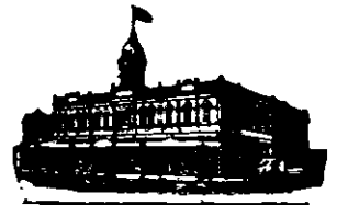
Te Aro House WELLINGTON
