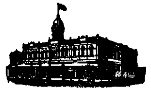
Te Aro House WELLINGTON
