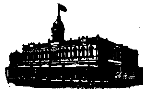
Te Aro House WELLINGTON
