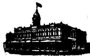
Te Aro House WELLINGTON
