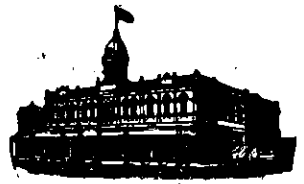
Te Aro House WELLINGTON
