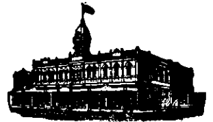
Te Aro House WELLINGTON
