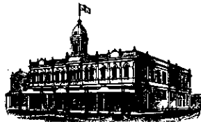
Te Aro House WELLINGTON
