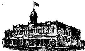
Te Aro House, WELLINGTON
