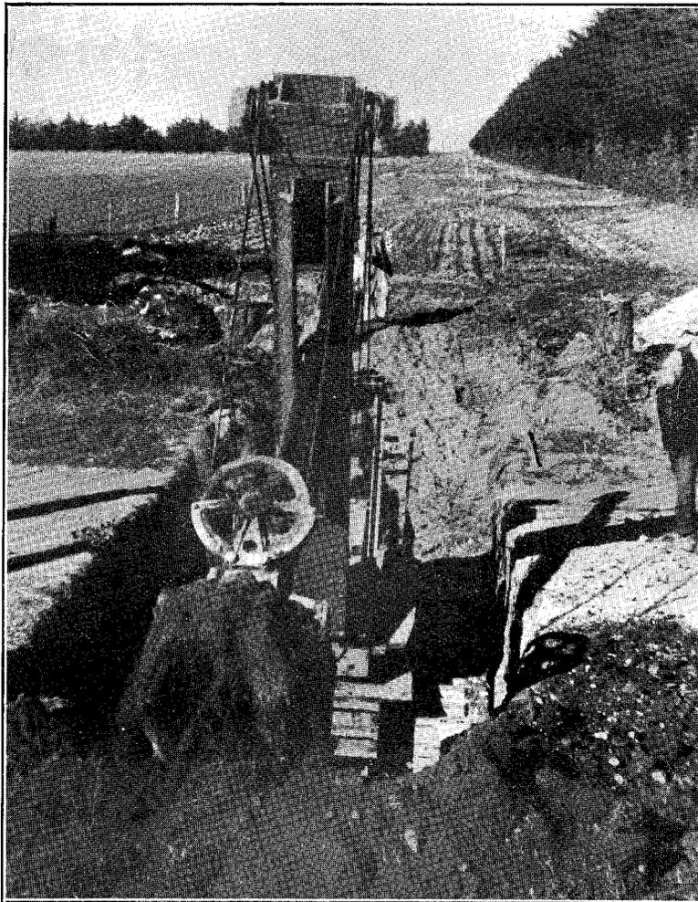
SPEEDER  $\frac{3}{8}$  YD. TRACTOR SHOVEL EXCAVATING SITE FOR ROAD-CROSSING SIPHON.
