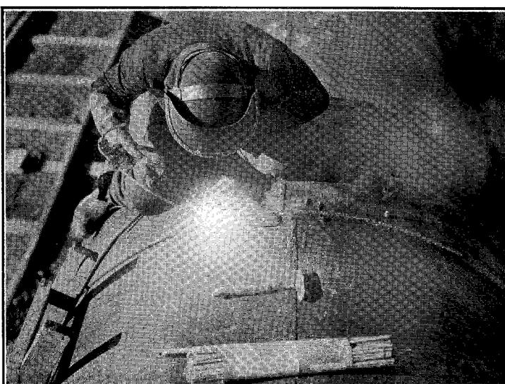
WELDING 6 FT.-DIAMETER STEEL PIPES.
