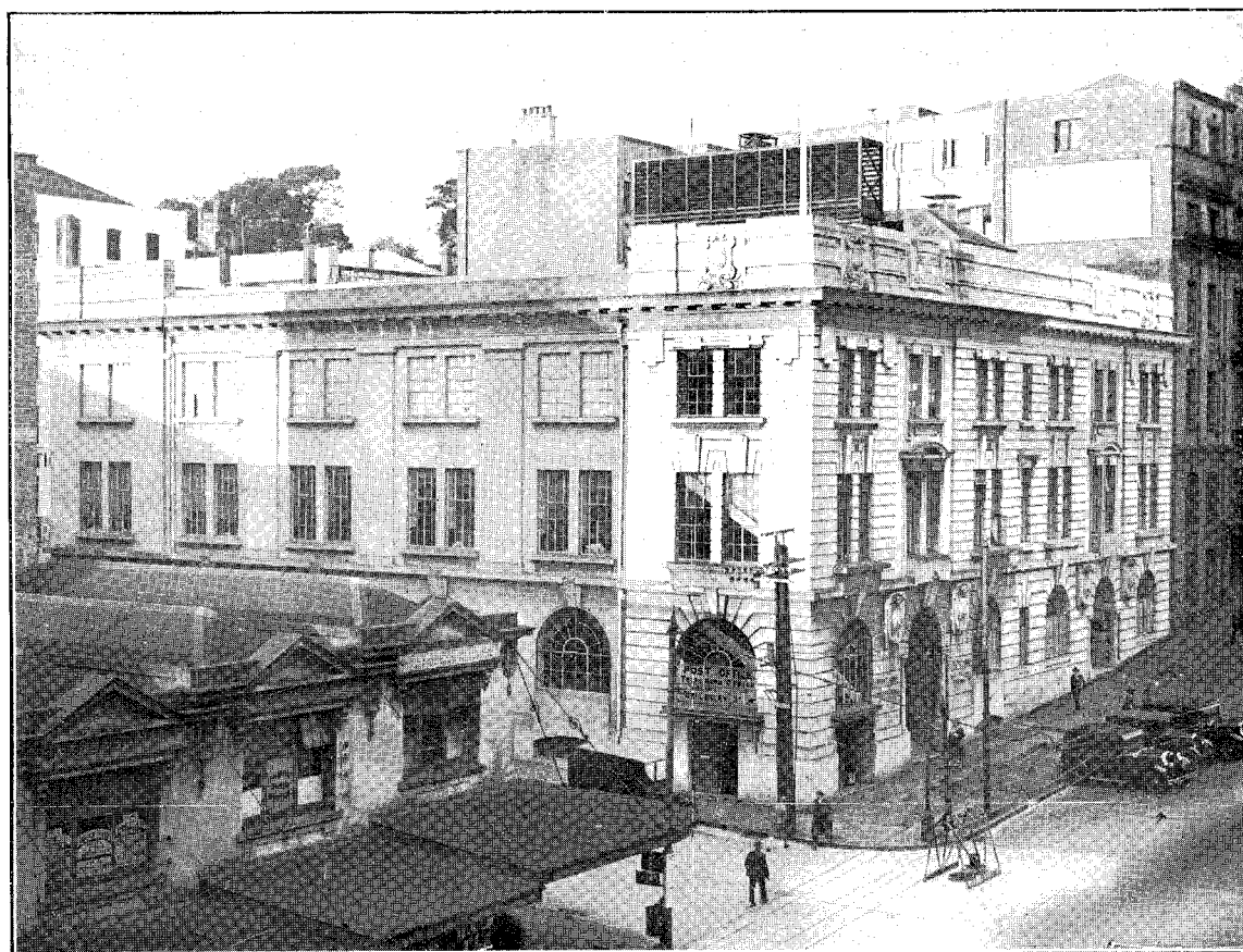
AUCKLAND: CENTRAL TELEPHONE EXCHANGE (INCLUDING RECENT ADDITION).
