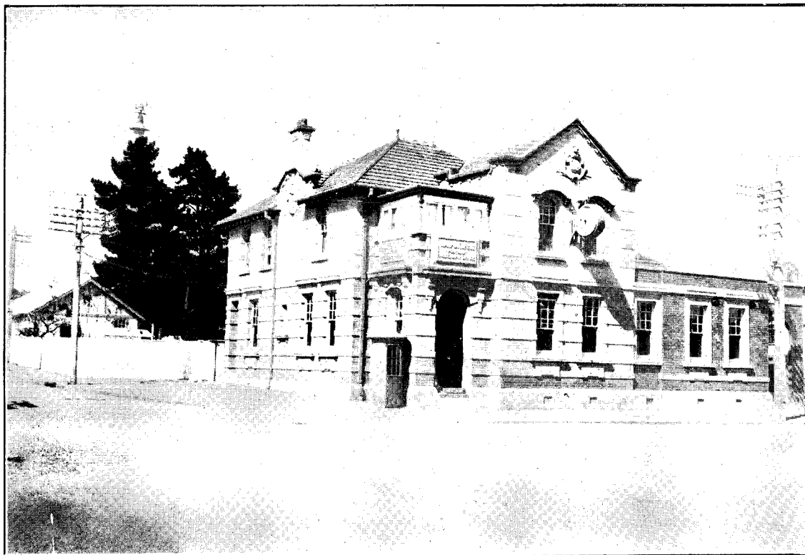
WAIPUKURAU POST-OFFICE BUILDING. (SHOWING RECENT ADDITION.)
