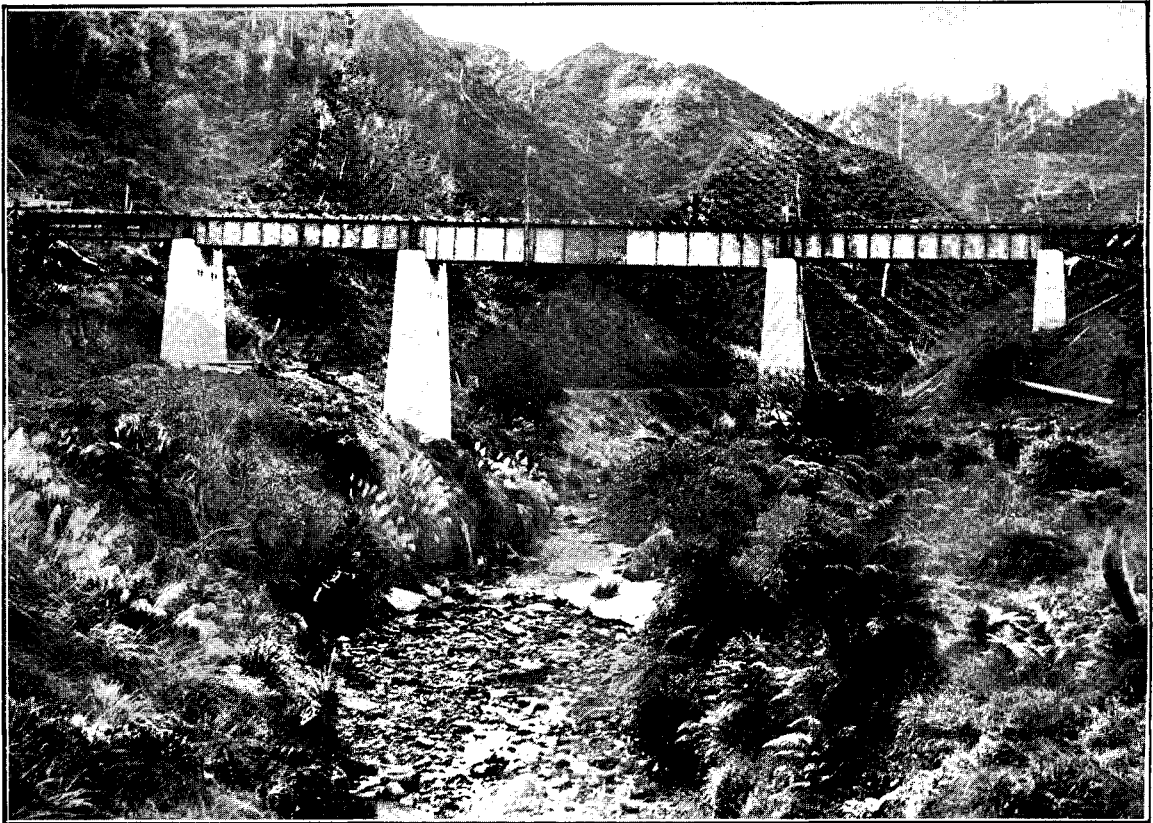
RAEKOHUA STREAM BRIDGE AT 49 M. 16 CH. One 60 ft., two 40 ft., one 30 ft., and one 25 ft. spans. STRATFORD - MAIN TRUNK RAILWAY.—WEST END.
