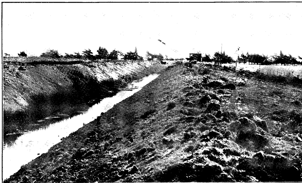
VIEW SHOWING CONDITION OF DRAIN AFTER WIDENING AND TRIMMING.
