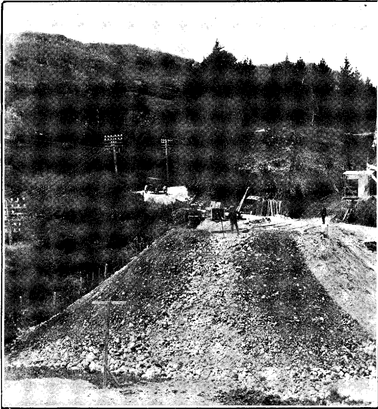
WELLINGTON NAPIER (VIA WAIRARAPA) MAIN HIGHWAY : CUTTING TO IMPROVE ALIGNMENT.
