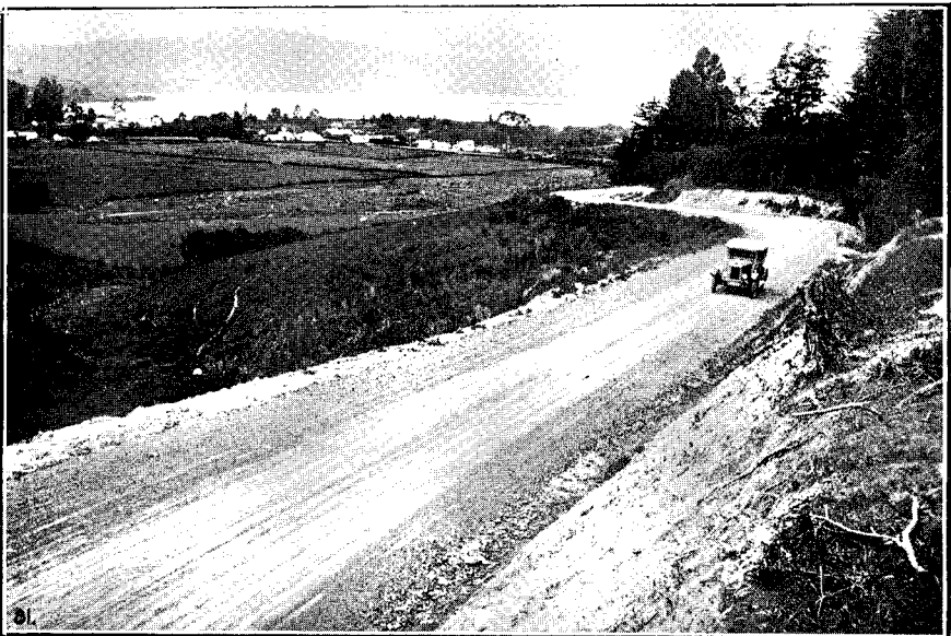
WATER-BOUND MACADAM BEFORE BEING SURFACE-TREATED WITH BITUMEN.
