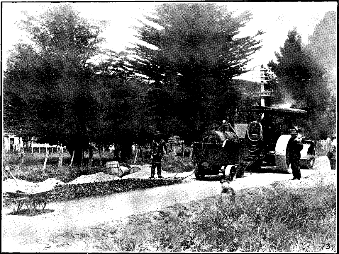
WELLINGTON-NAPIER (VIA WAIRARAPA) MAIN HIGHWAY, AKATARAWA SECTION: CONSTRUCTION OF BITUMINOUS-MACADAM WEARING-SURFACE.
