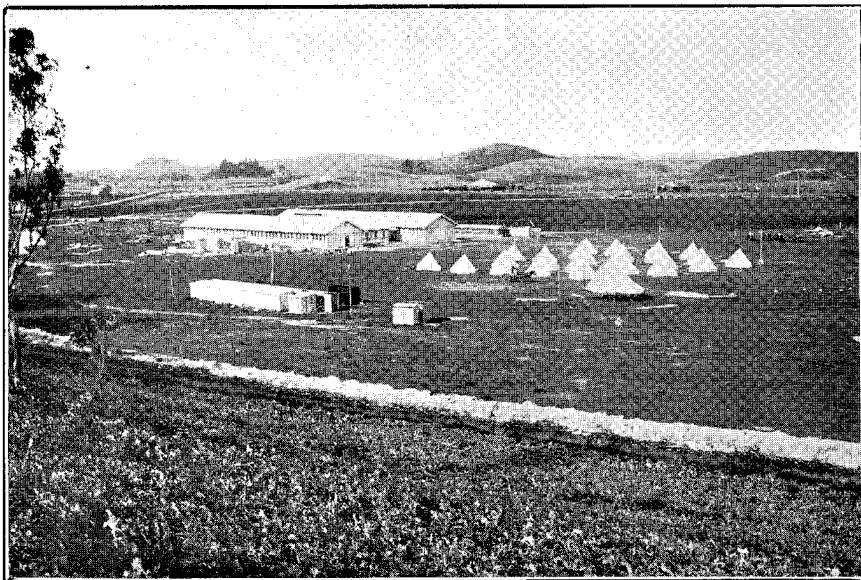
GENERAL VIEW OF BUILDINGS.
