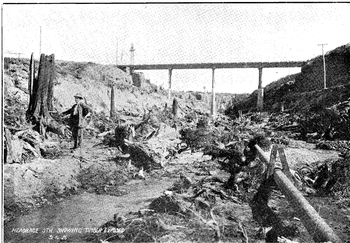
ARAPUNI HYDRO-ELECTRIC-POWER DEVELOPMENT : HEAD-RACE, SHOWING BURIED TIMBER.
