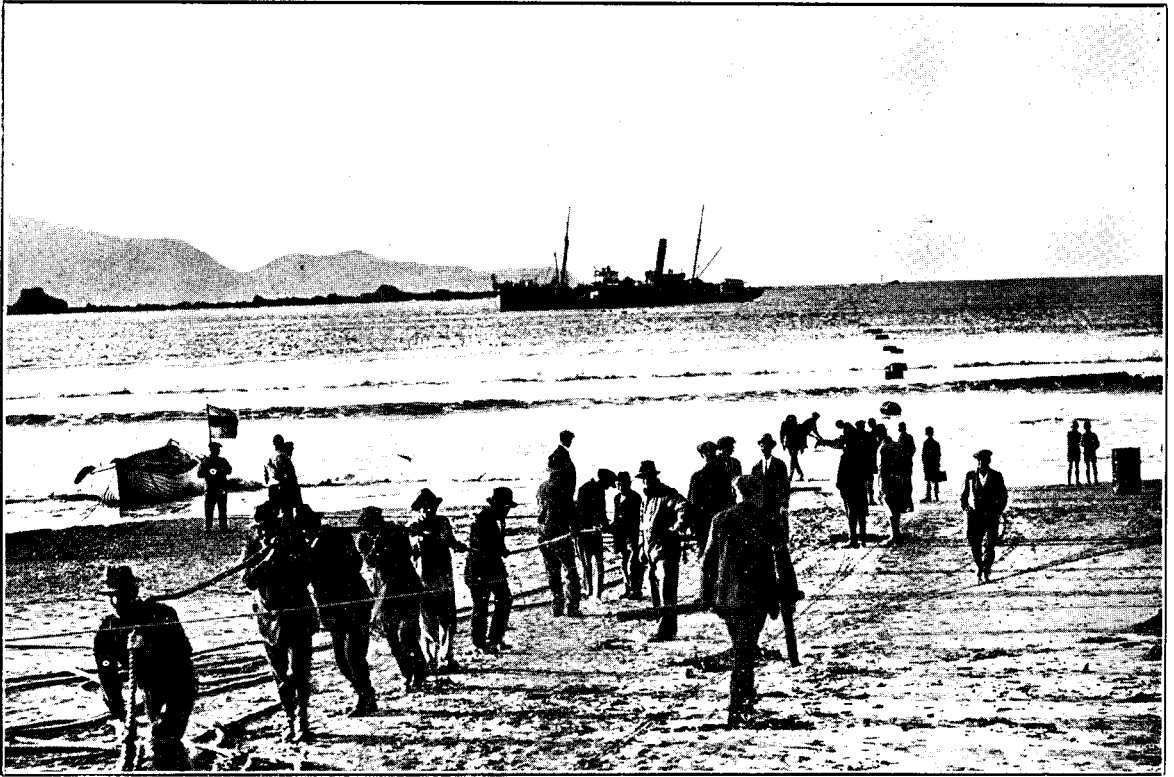
HAULING-IN SHORE END OF CABLE AT LYALL BAY.
