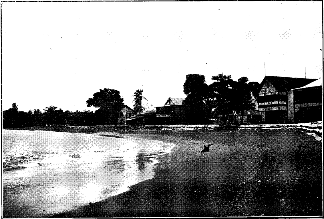
SEA-WALL, APIA, UNDER CONSTRUCTION, JANUARY, 1926.
