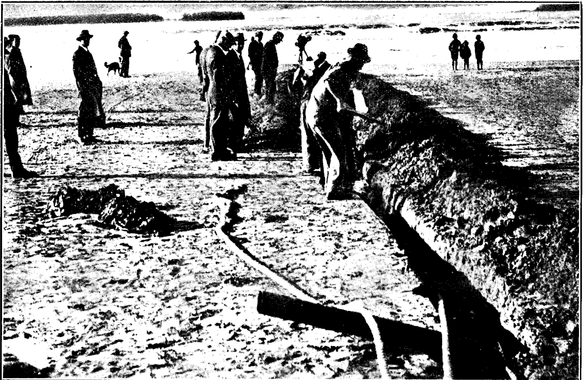
PREPARING TRENCH FOR SHORE END OF CABLE AT LYALL BAY.
