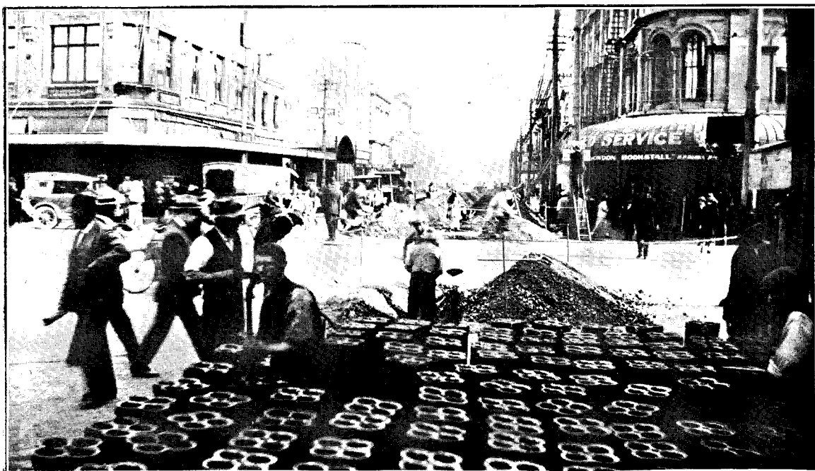
LAYING DUCTS FOR UNDERGROUND TELEPHONE-CABLES, HEREFORD STREET, CHRISTCHURCH.
