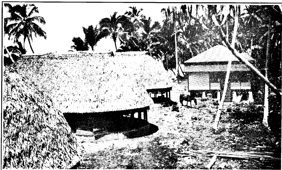
FIG. 11. District Hospital at Lalomamu, in the Meipata district. This photograph was taken on completion of the buildings, before the grounds had been cleaned up.
