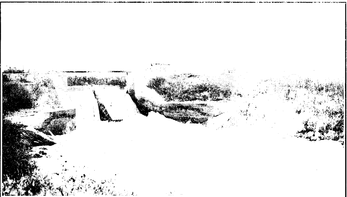
TYPES OF OVERFALLS ON DITCHES.
