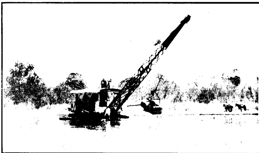
WALKING DRAG-LINE EXCAVATOR.
