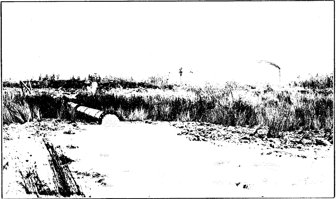
WAIHOU DREDGE. OUTLET END OF DISCHARGE PIPE.
