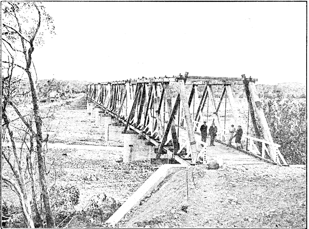
ROAD BRIDGE OVER HAPUKA RIVER, KAIKOURA COUNTY.
