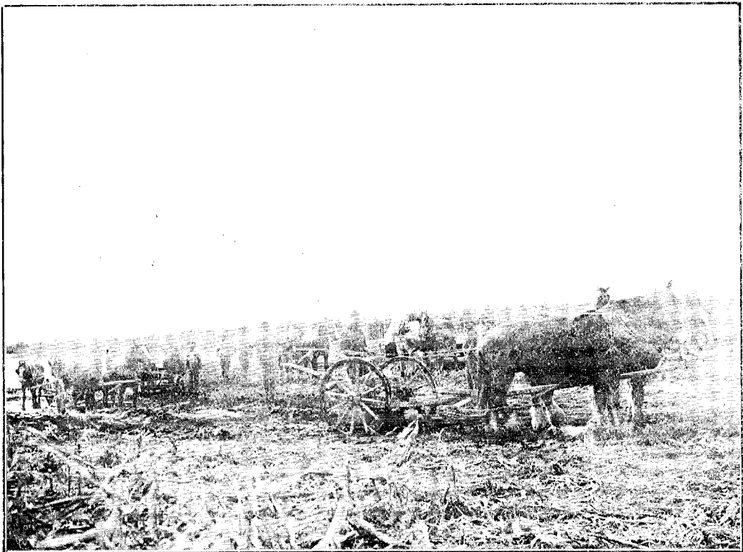
WHEEL SCOOPS AT WORK ON OMEHU OUTFALL.
