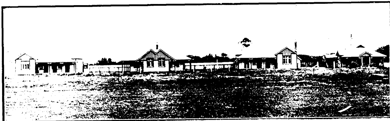
LIVING ACCOMMODATION PROVIDED FOR FLAX-MILL WORKERS, MASSACHUSETTS (WILSON & FLAX MILLING COMPANY).
