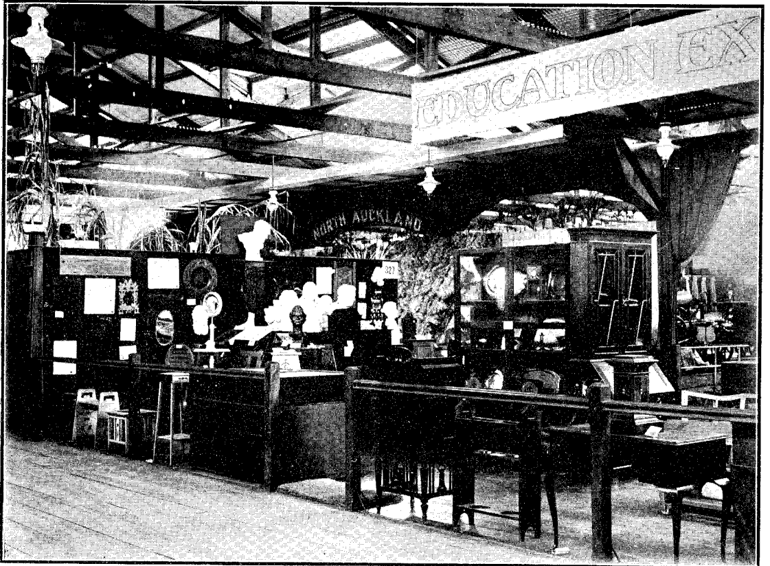
CABINETMAKING AND APPLIED ART BAY.
