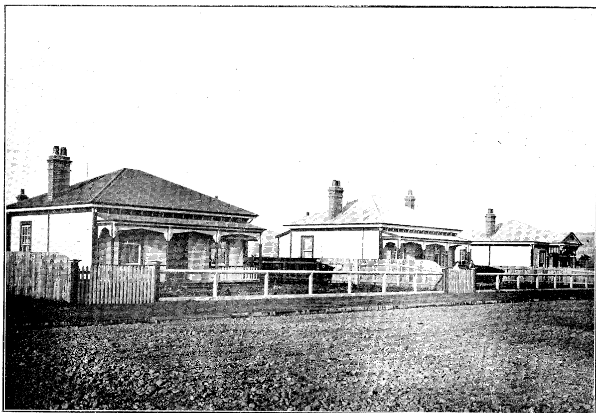
LOUGHNAN SETTLEMENT, PALMERSTON NORTH.
