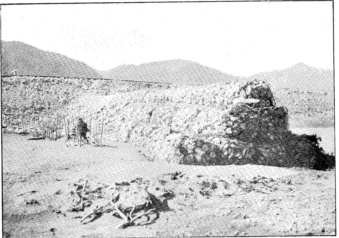
MIDLAND RAILWAY.—PROTECTIVE GROUYNE, WAIMAKARIRI RIVER.
