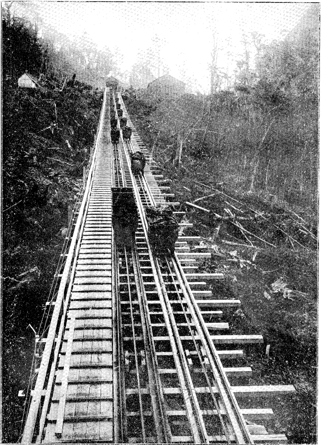
LIVERPOOL STATE COLLIERY, GREYMOUTH. - VIADUCT APPROACHING MIDDLE HYDRAULIC BRAKE ON MAIN ENDLESS-ROPE GRAVITATION-HAULAGE INCLINE.
