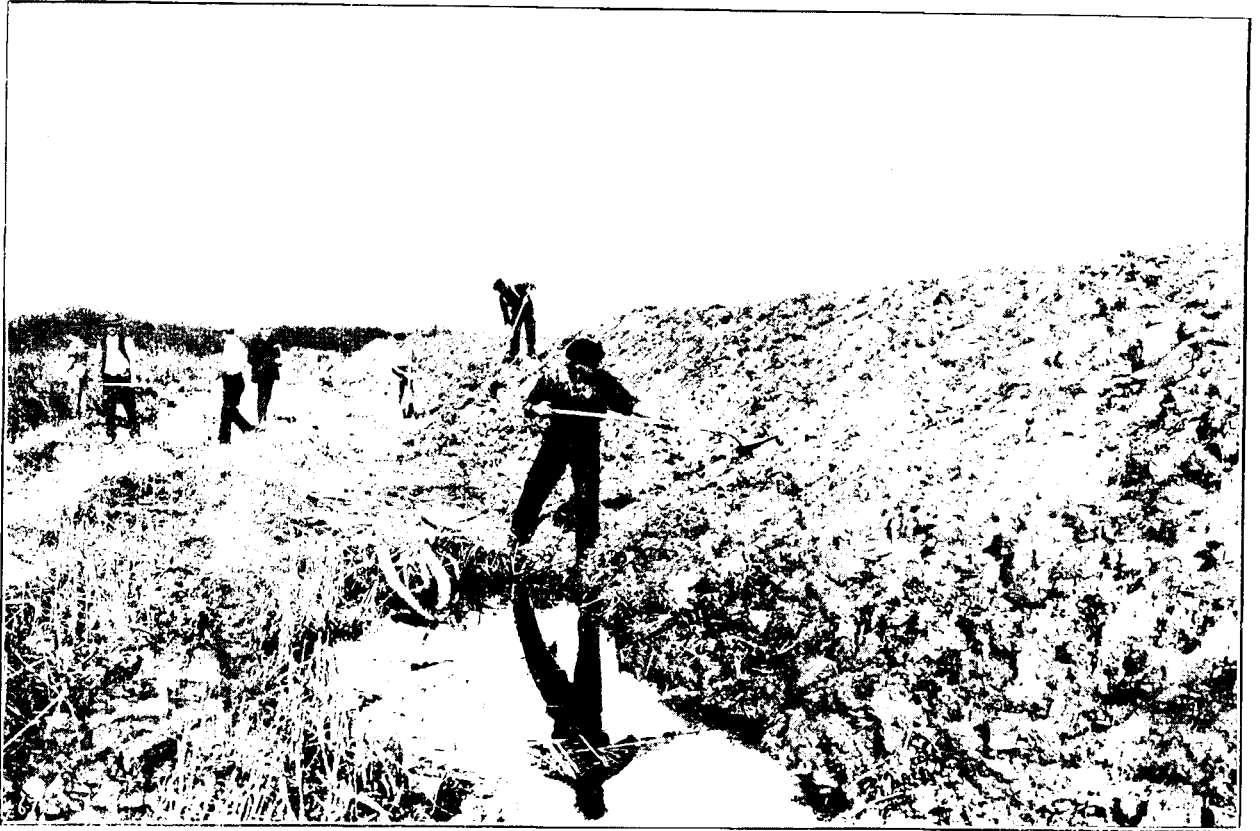
COMPLETING STOP BANK
