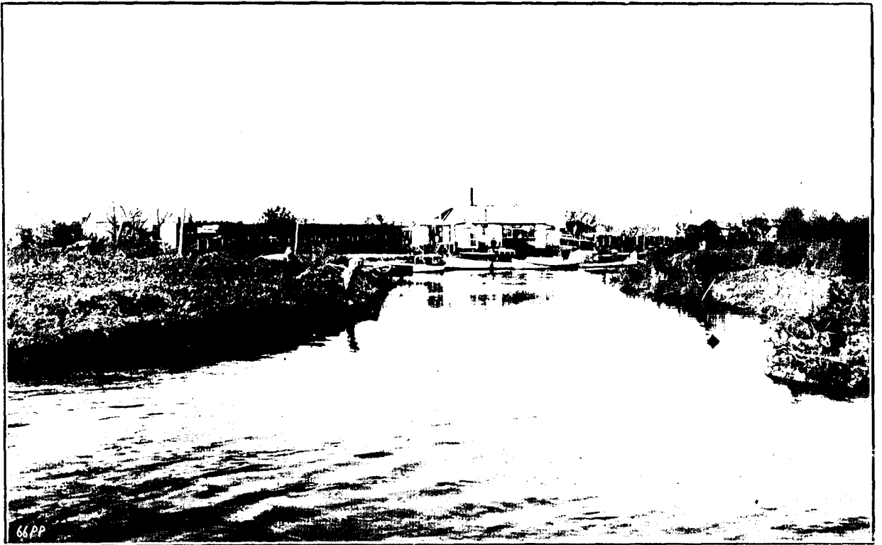
JUNCTION OF PIKAO RIVER AND AWALLI STREAM, THE LATTER NOW BEING DREDGED AND WIDENED.
