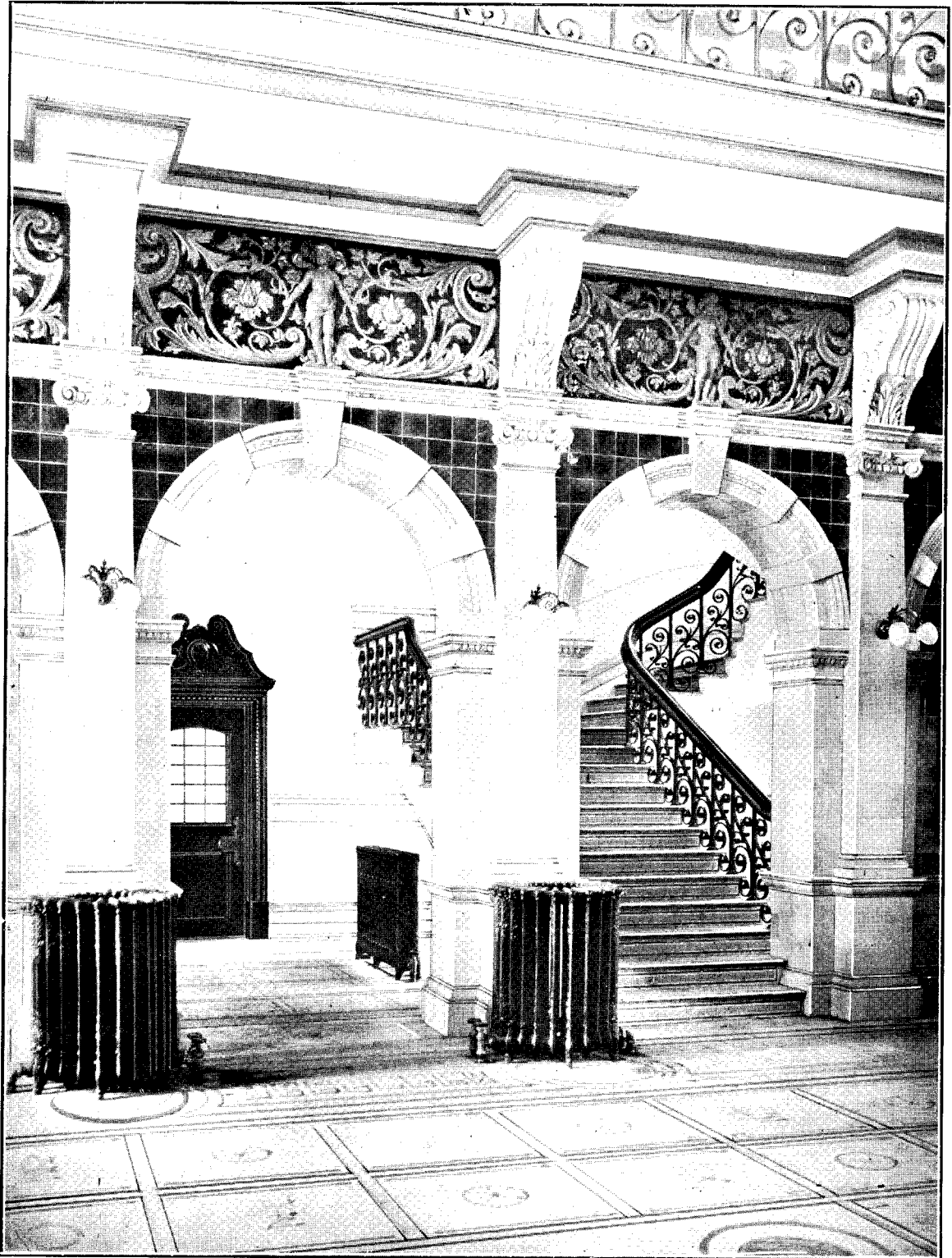
STAIRCASE, DUNEDIN RAILWAY-STATION.
