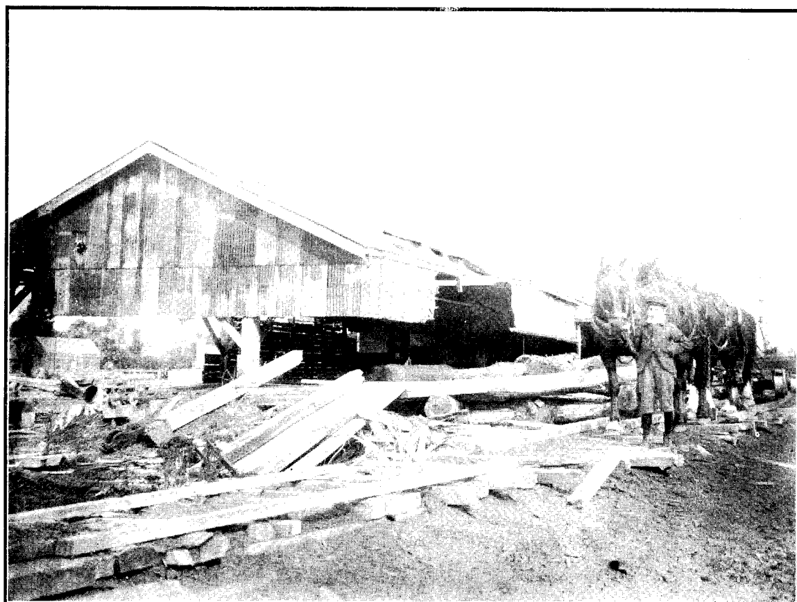
No. 23.] McCALLUM AND Co.'s MILL AT COLAC, SOUTHLAND.
