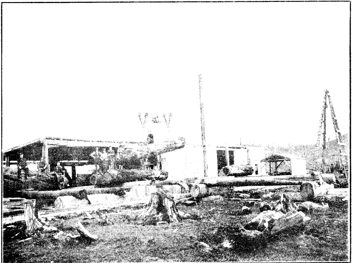
[No. 18.] — OVERHEAD APPARATUS FOR HAULING LOGS, NAAPAHUHI, HAWAIIAN ISLANDS.
