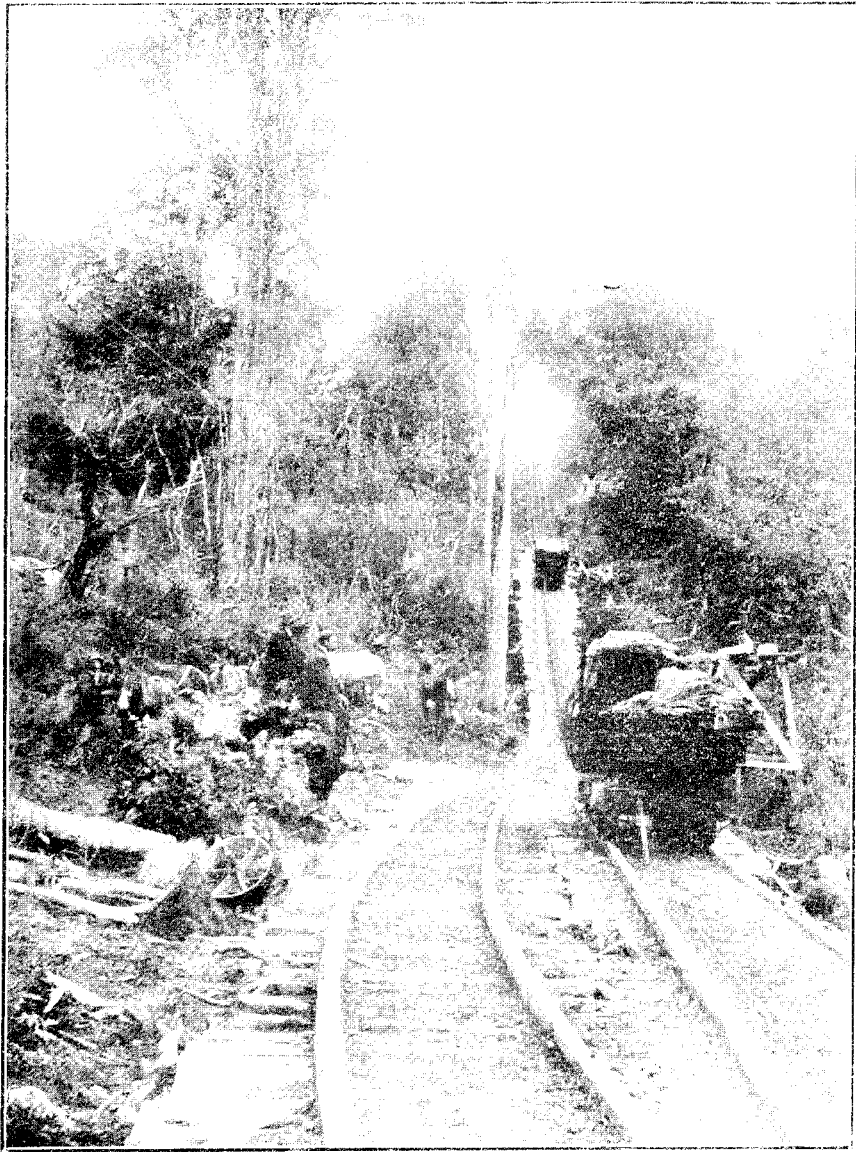
[No. 17.] — HAULING TIMBER TO SHIP EXPOSED, OREGON, HAWAIIAN ISLANDS.
