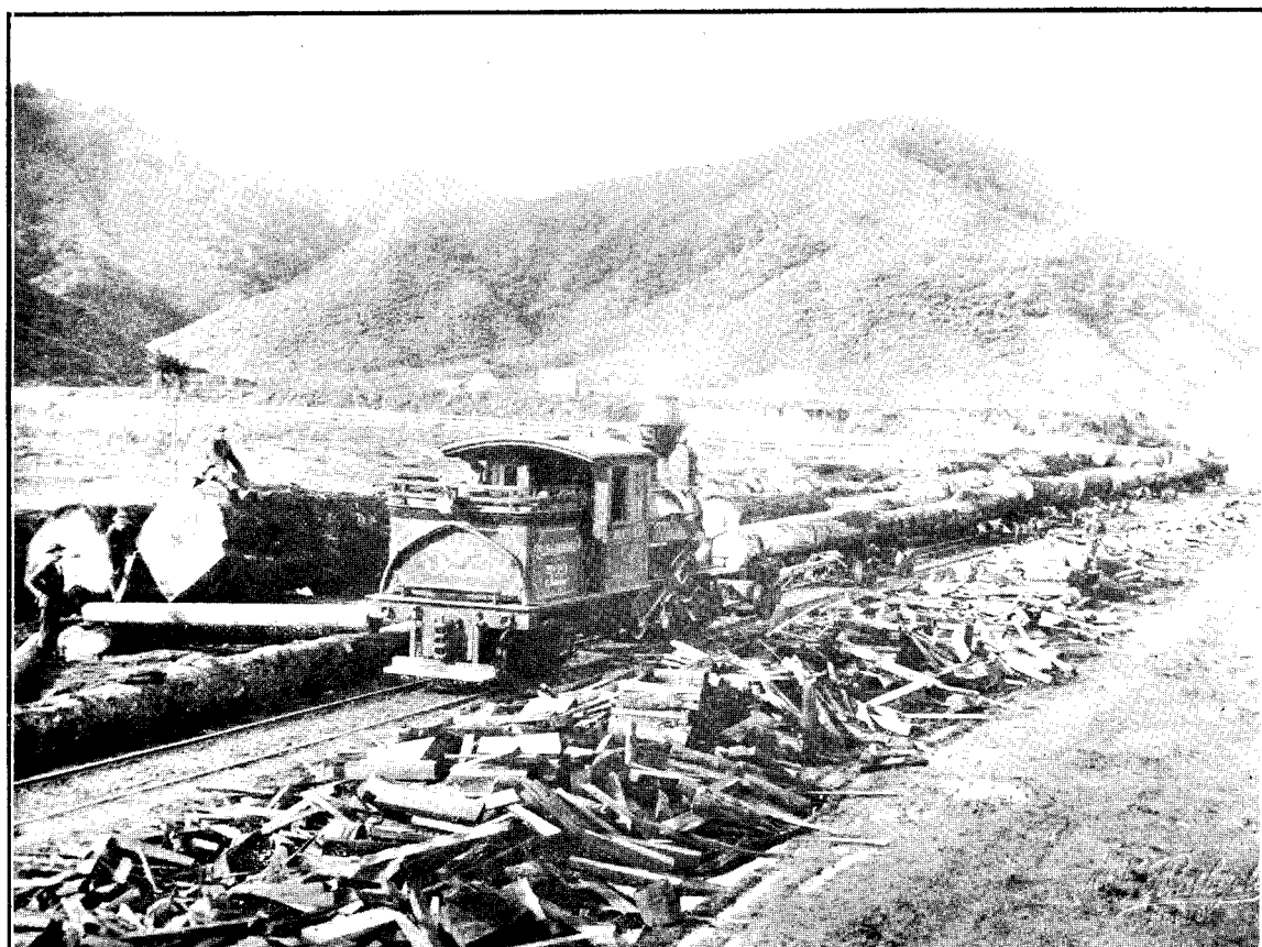
No. 14.] ENGINE HAULING LOGS AT MANGAPEHI, TARANAKI.
