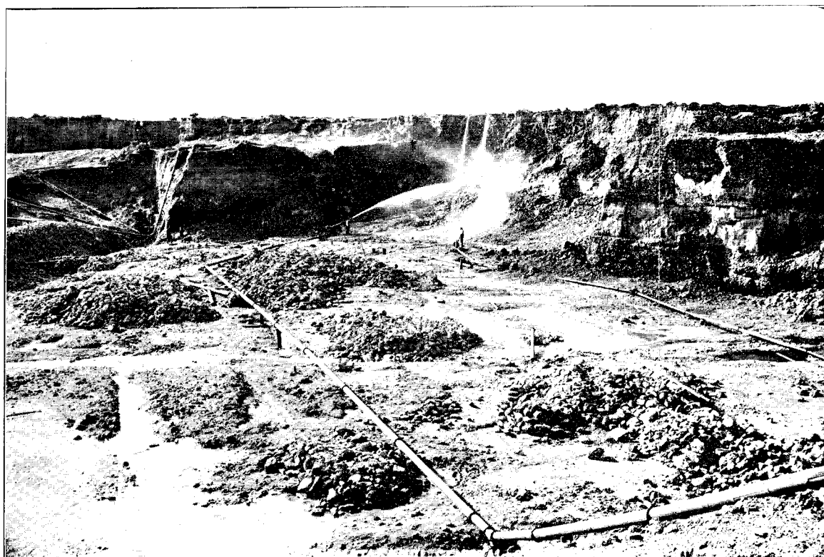
UNDAUNTED GOLD-MINING COMPANY'S CLAIM, MATAKANUI, OTAGO. SLUICING AND ELEVATING.
