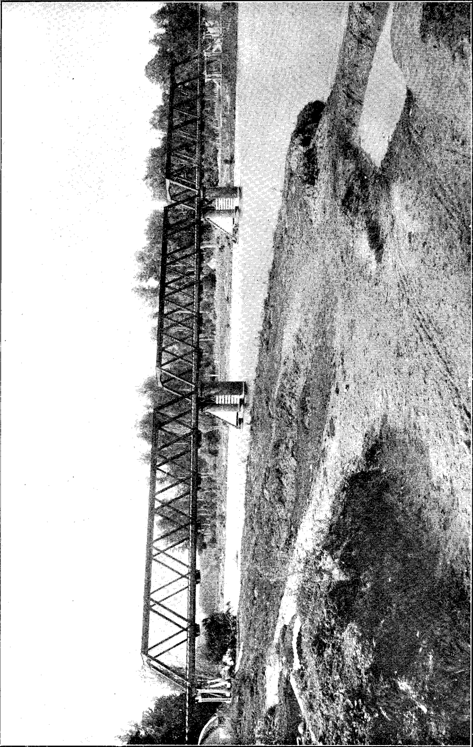
NORTH ISLAND MAIN TRUNK RAILWAY: COMBINED ROAD AND RAILWAY BRIDGE OVER WANGANUI RIVER NEAR TAUMARUNGI. Five 20 ft. timber, and three 122 ft. 6 in. steel spans, on timber and braced cylinder piers; total length, 472 ft.
