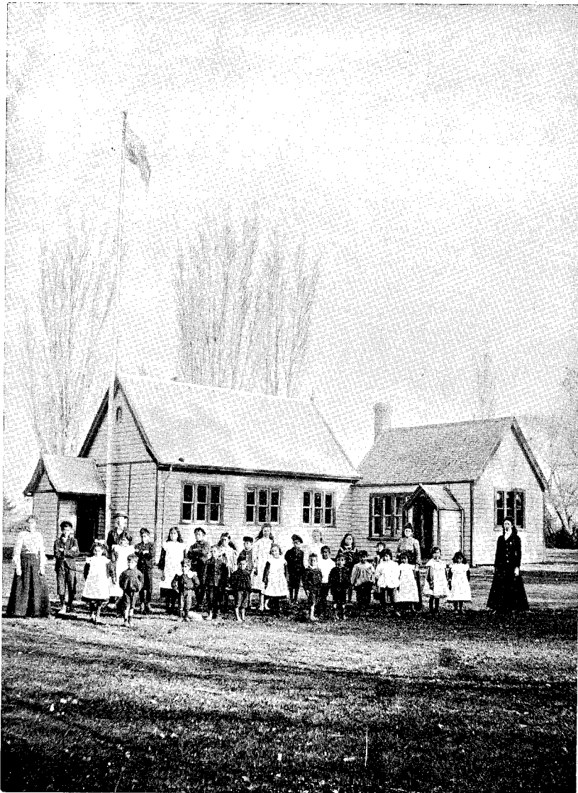
A South Island School, Kaiapoi.
