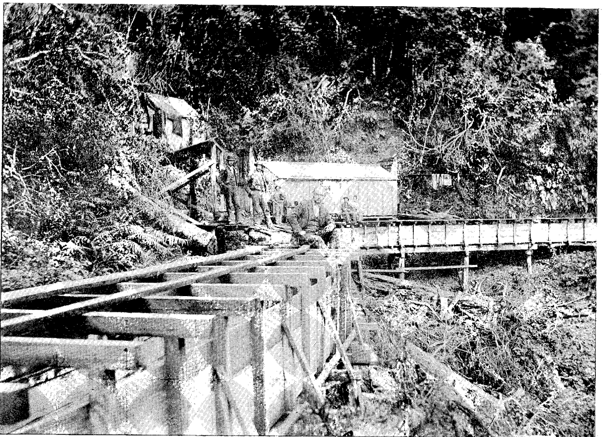
Waiwhero Sluicing and Dredging Company (Limited) : Main Canoe Creek Water-race, thirty-five heads capacity, six miles and a half long.
