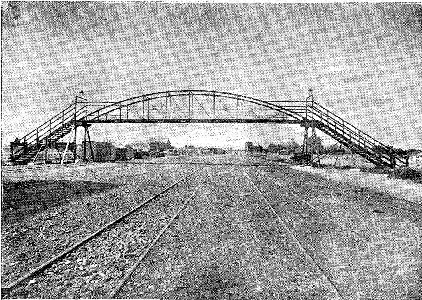
Feilding Overbridge (built of old rails); span 77 ft. Cost £333.
