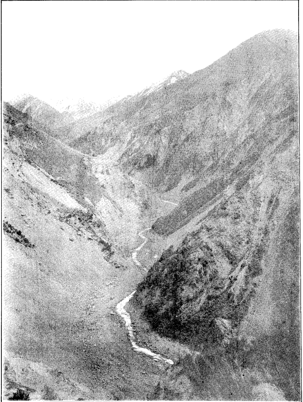
PHOTO LITHOGRAPHED AT HEAD OFFICE, LAMES & SIBBIE (N.Z.) WELLINGTON N.Z. 1901 Midland Railway, Mount Torlesse Section, Staircase Gully: View looking up gulley from bridge-site.
