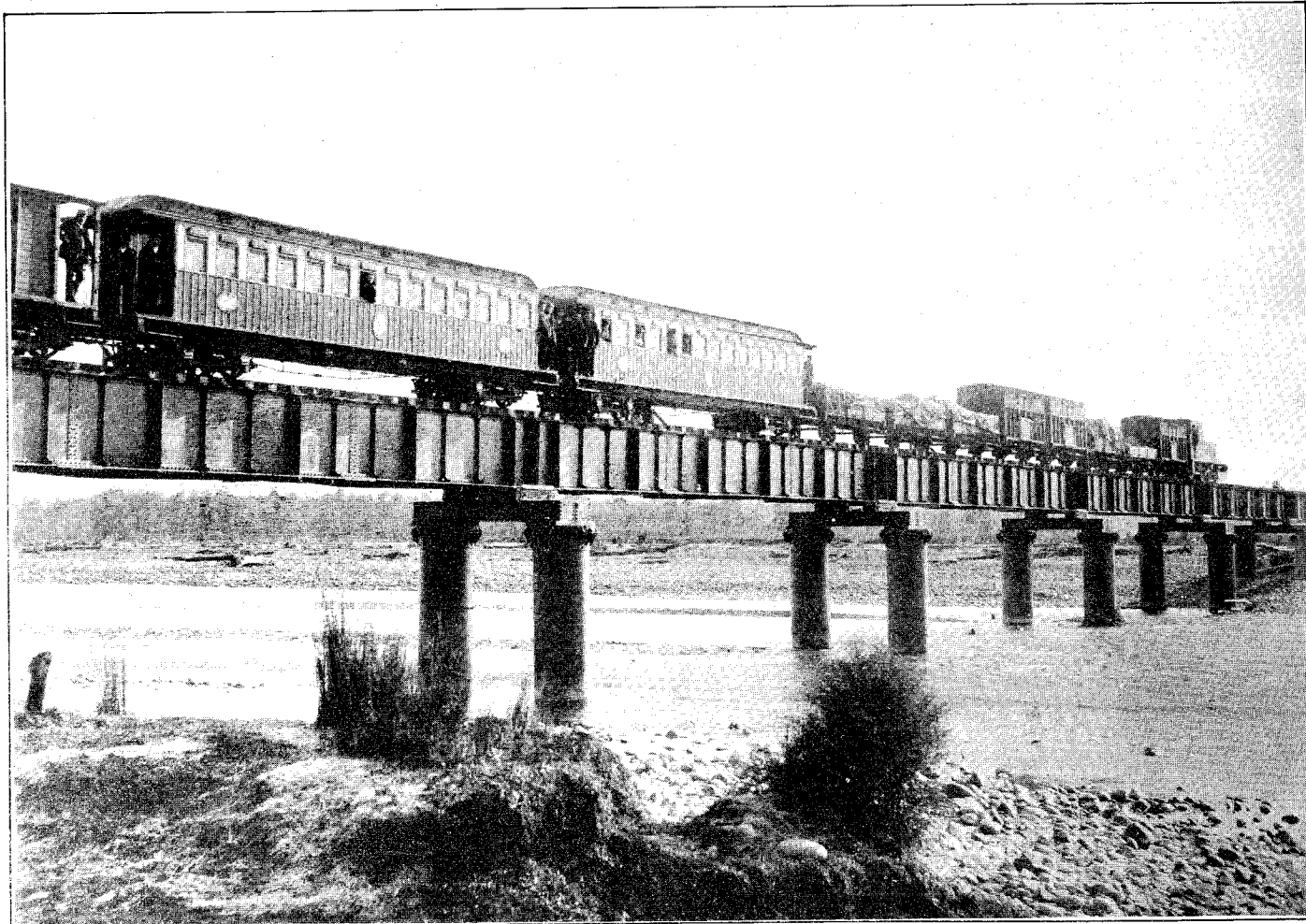
Midland Railway, Bridge over Little Grey River: Ten spans of 66 ft., and three of 11 ft.; total length of cylinders, 33 ft.
