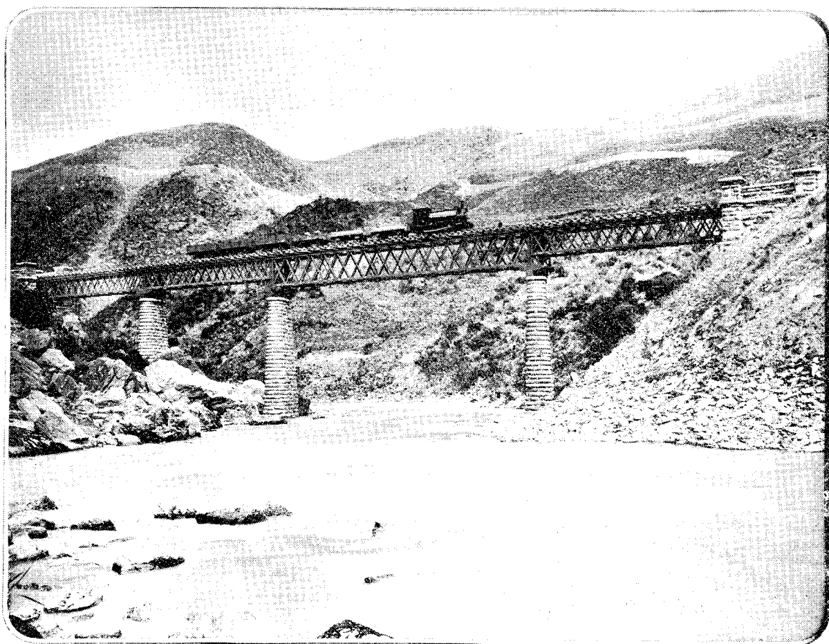
Otago Central Railway.—Bridge over the Taieri River at 16 miles 20 chains.
