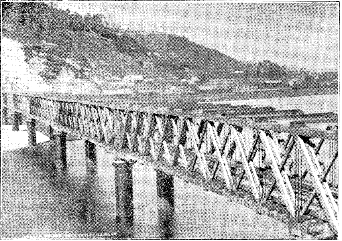
Cobden Bridge—over Grey River. 6 spans of 109ft. Height from bed of river to road level, 43ft.
