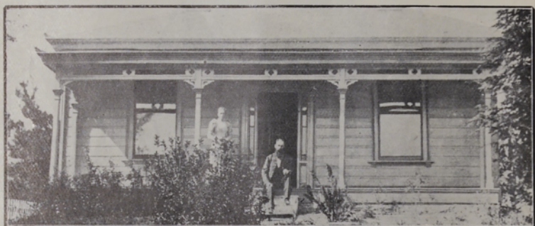
THE MANSE, TUAPEKA WEST
