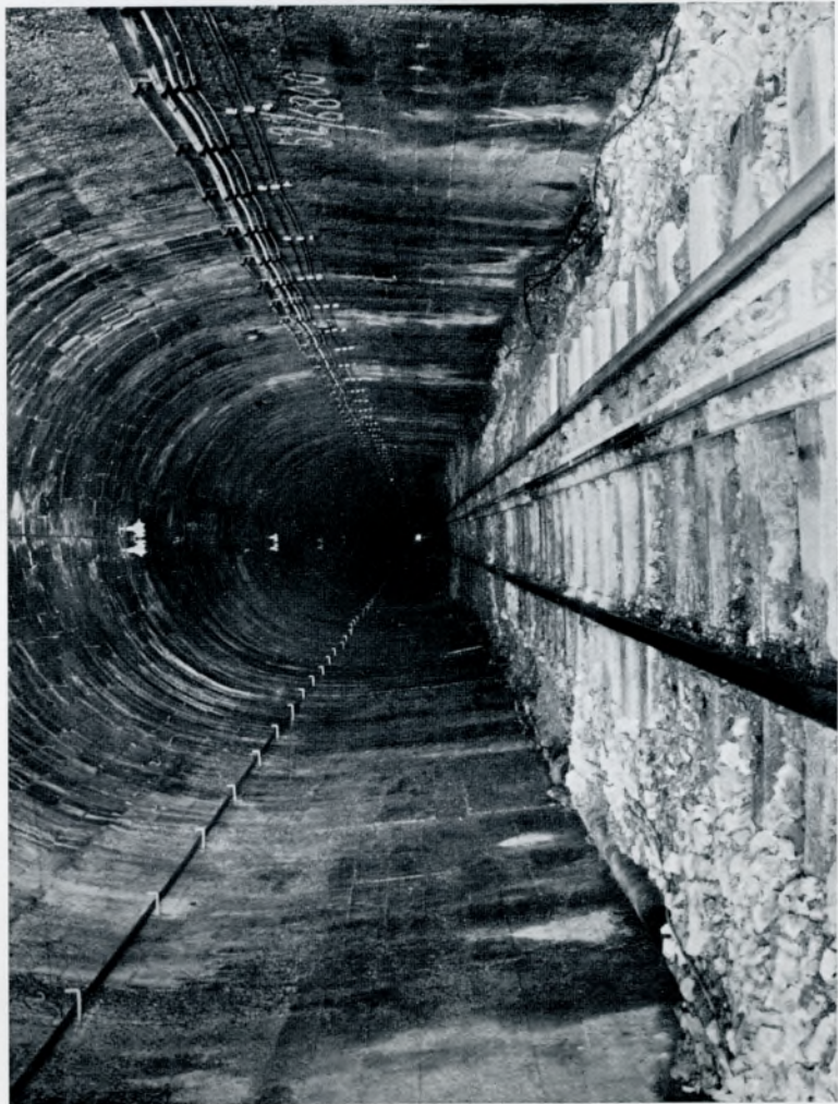
FIVE AND A QUARTER MILES OF TUNNEL, LOOKING TOWARDS OTIRA
