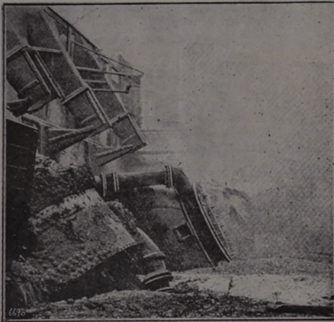
THE CONVERTER TURNED UP, WITH THE "BLOW" IN OPERATION.
