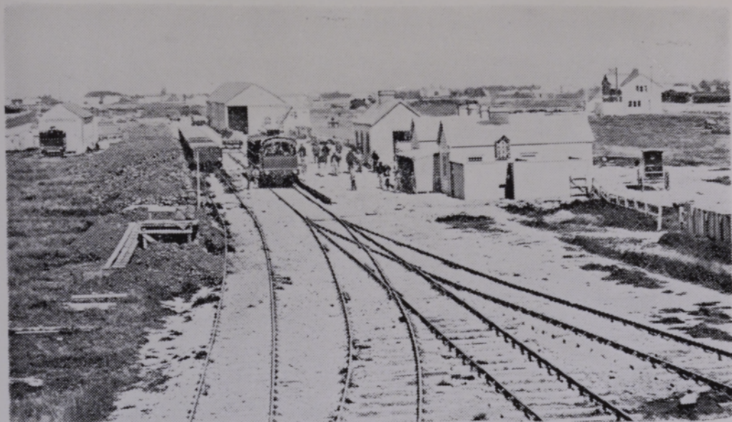
The first Christchurch Station in 1863, situated near Madras Street. Note broad gauge track, loco. and stock, also three-way points.
